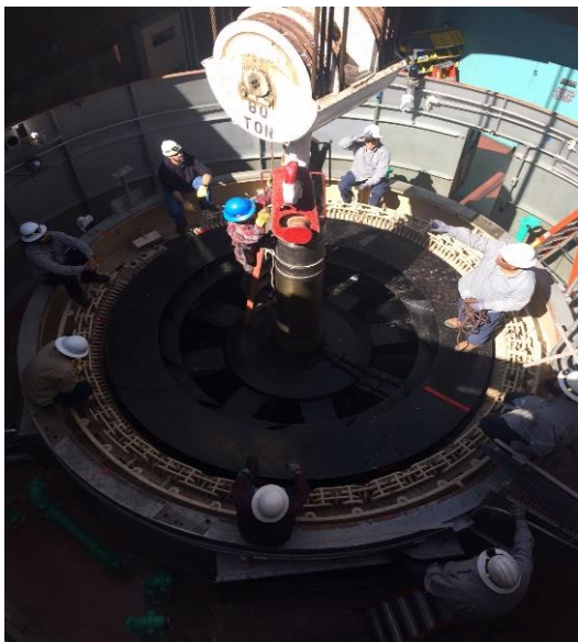
Prepping JU-6 Rotor for Removal
