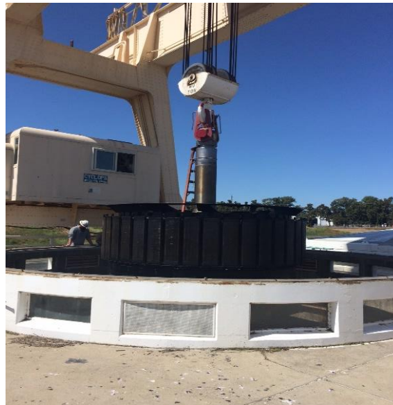
JU-6 Rotor Removed
